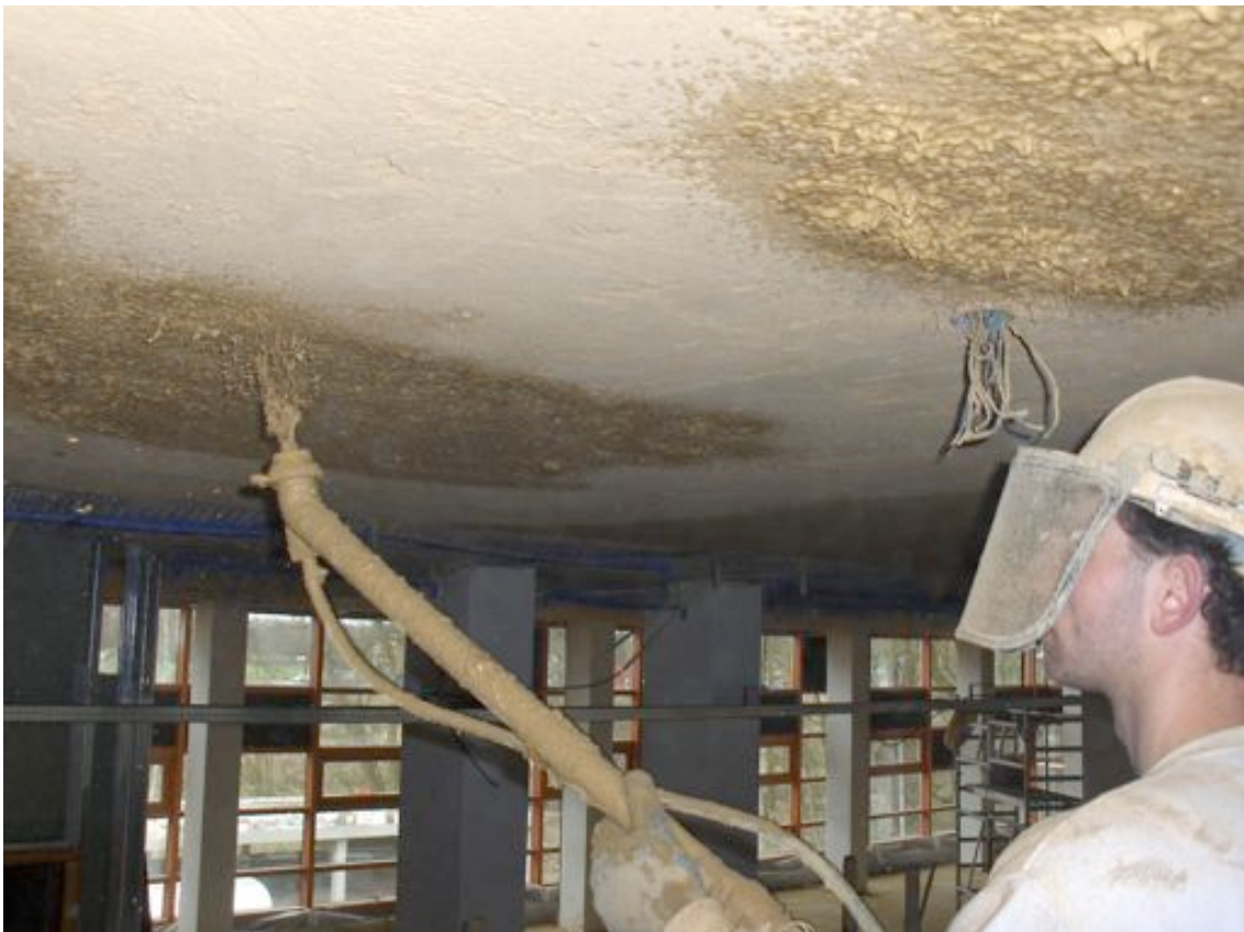
Photo 2 – Spraying clayplaster WWF Zeist, the Netherlands. (credits: Michel Leeman)
