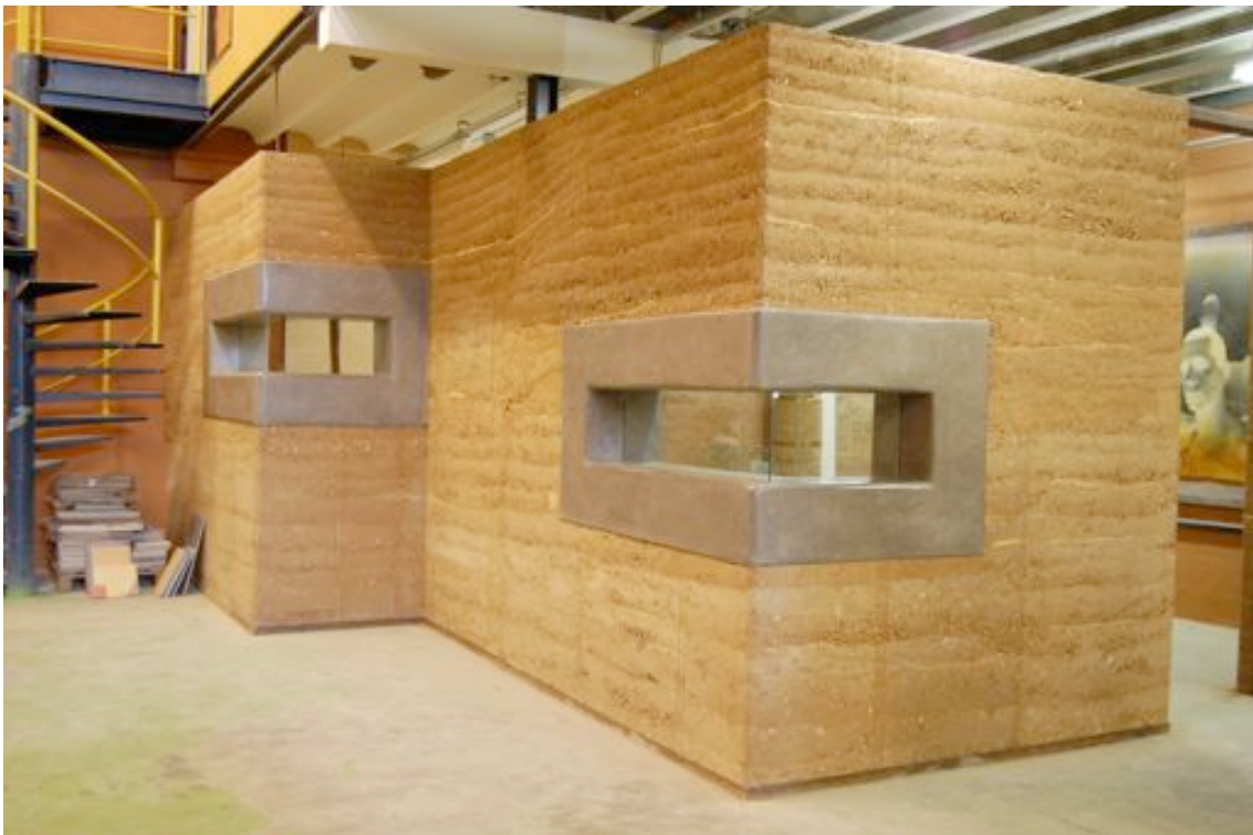
Photo 5 – Office Amsterdam, the Netherlands (credits: Leemwerk)
